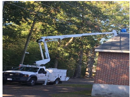
Focus Communications installing new cameras.
